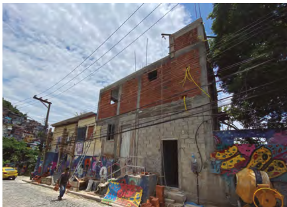
Sede da Rede NAMI durante a reforma. NAMI headquarters during renovation.
